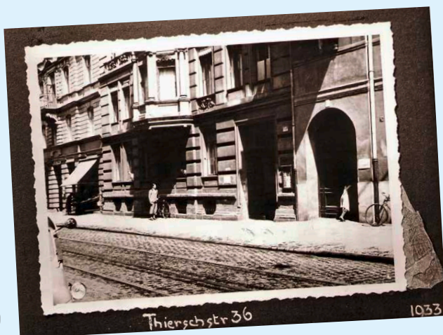
Fig. 1: The history of Rohde & Schwarz started at 36 Thierschstraße in Munich.
